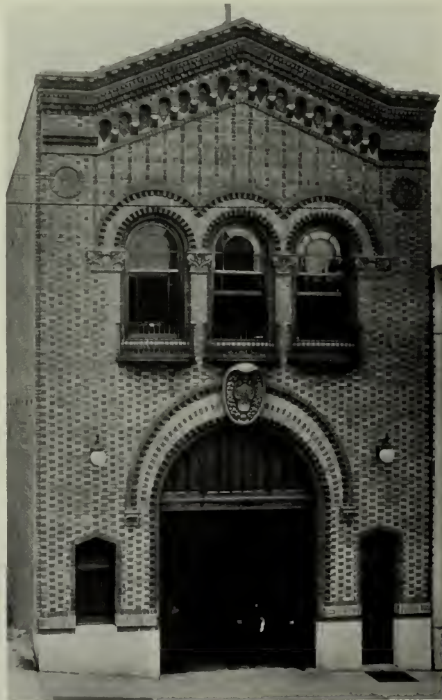
ENGINE HOUSE NO. 41. Loring P. Rixford, City Architect.
